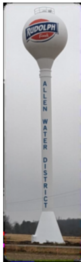
Rudolph Foods Water Tower
