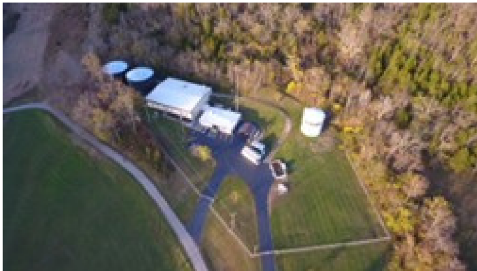
ACRWD Water Treatment Plant aerial view
